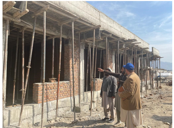
Construction of Laghman infectious diseases ward.
