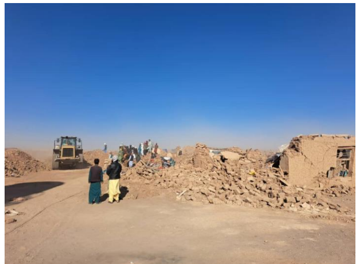
Photo 1: Most of homes were completely destroyed. The search and rescue operation continues in Zindajan district, Herat Province.
