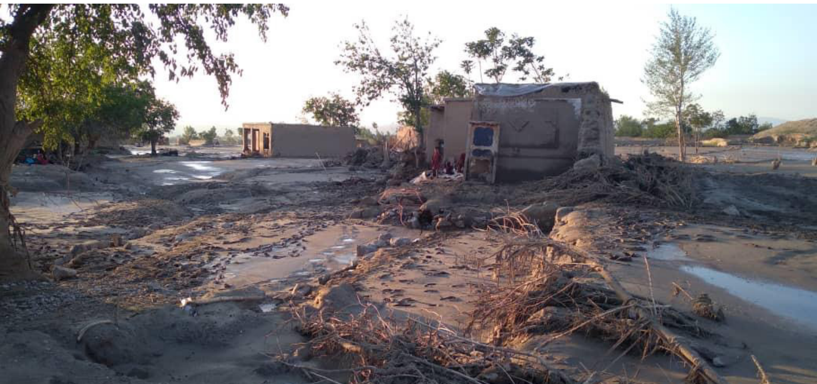
Damaged infrastructure in flood-affected communities. © WHO
