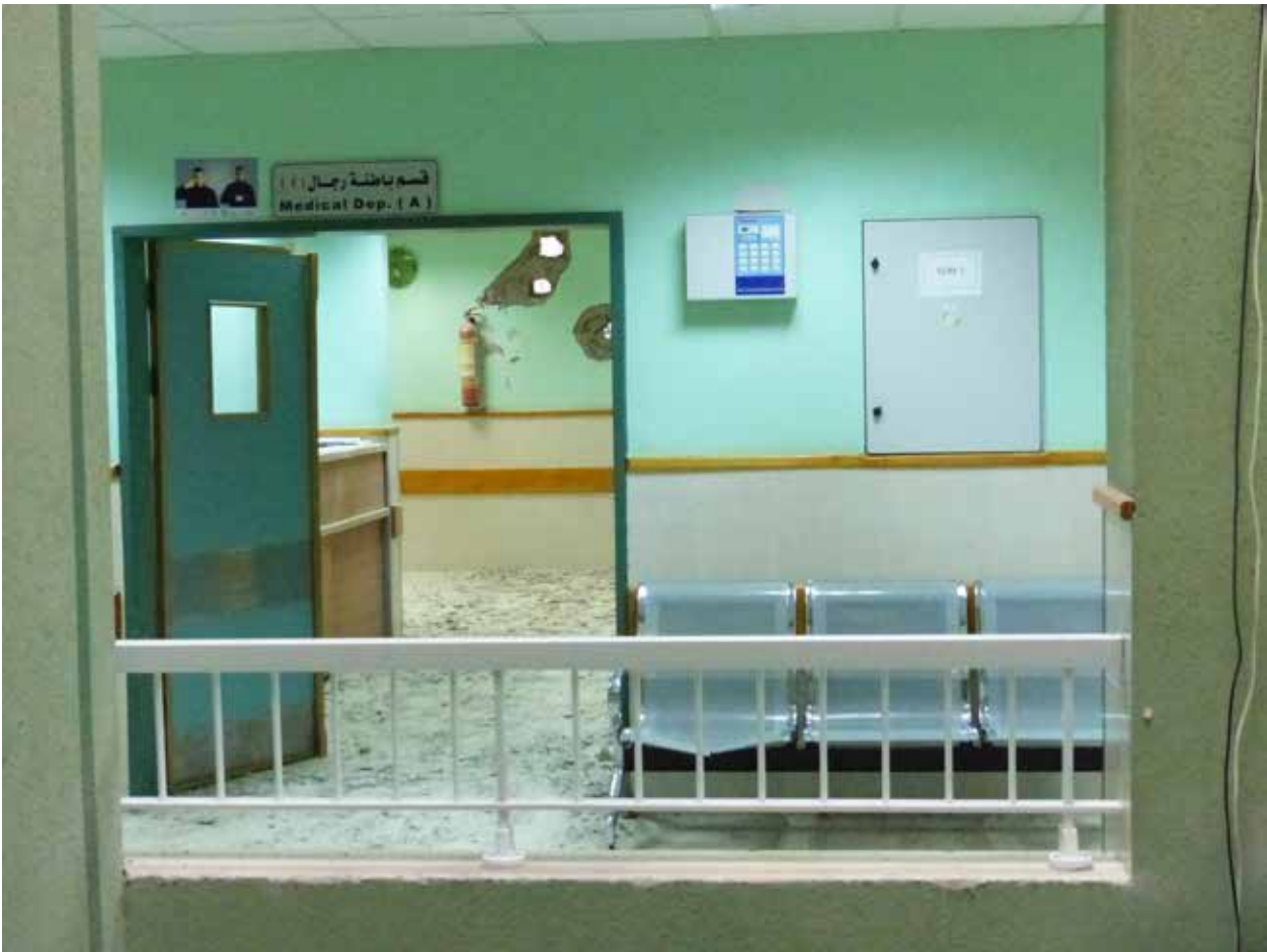
Al-Aqsa hospital, a Ministry of Health facility in Gaza, hit by rockets on 21 July 2014 © WHO
